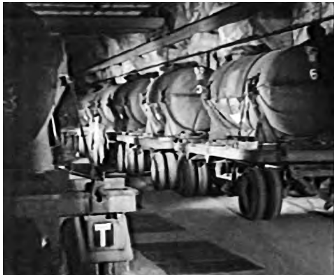
Road tankers for holding Runcol or Pyro in the Rhydymwyn tunnels during the war. Photo from Valley History Society
